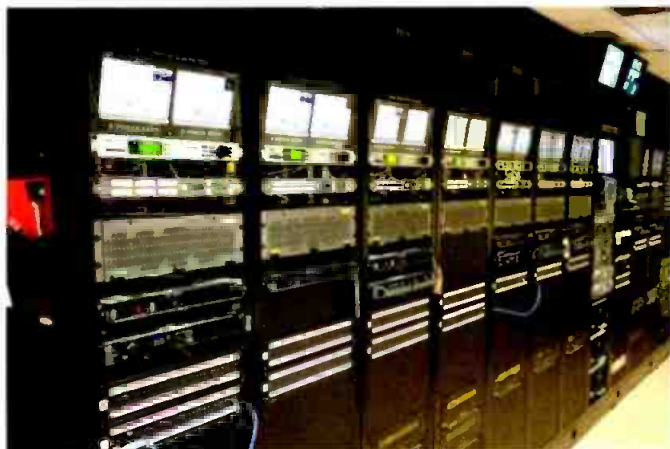
The network went with a traditional master control platform, with a Vizrt graphics engine and Evertz EQX ports for each channel physically mounted in individual racks to ensure channel redundancy.
